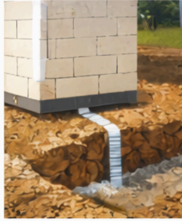
Barrier Formation – Creates a continuous treated zone
